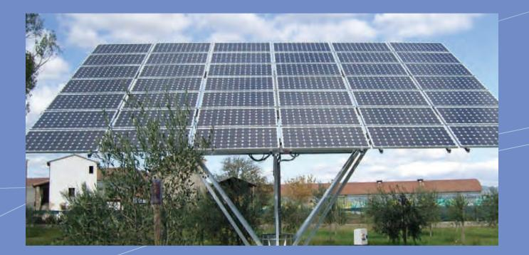
Location : Ancona, Italy Installation Date : June,2009 Application Type : Commercial System Size : 10KW Installation Type : Ground Mounted & Tracker System Module Supplier : Suntellite
